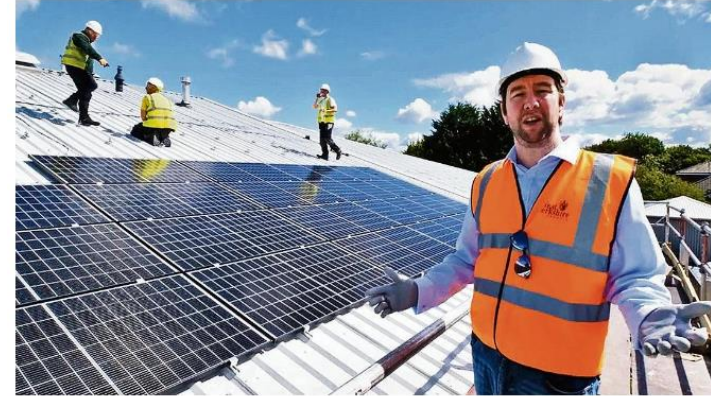
The Phoenix Centre in Newbury is one of six sites where solar panels are being installed with the help of local investment YOUTUBE
