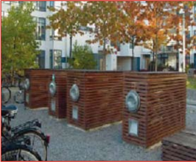
Communal storage facilities for each floor
