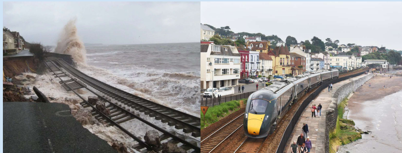
Dawlish Railway: Before and after repairs, 2014
