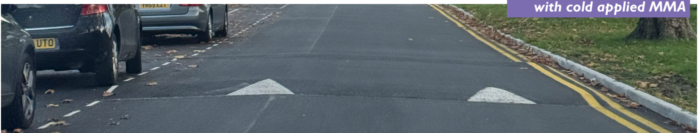
Figure 14: Pinehurst Avenue with cold applied MMA
