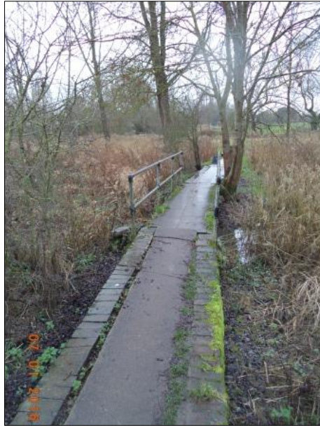
Deteriorated causeway and bridge crossing
