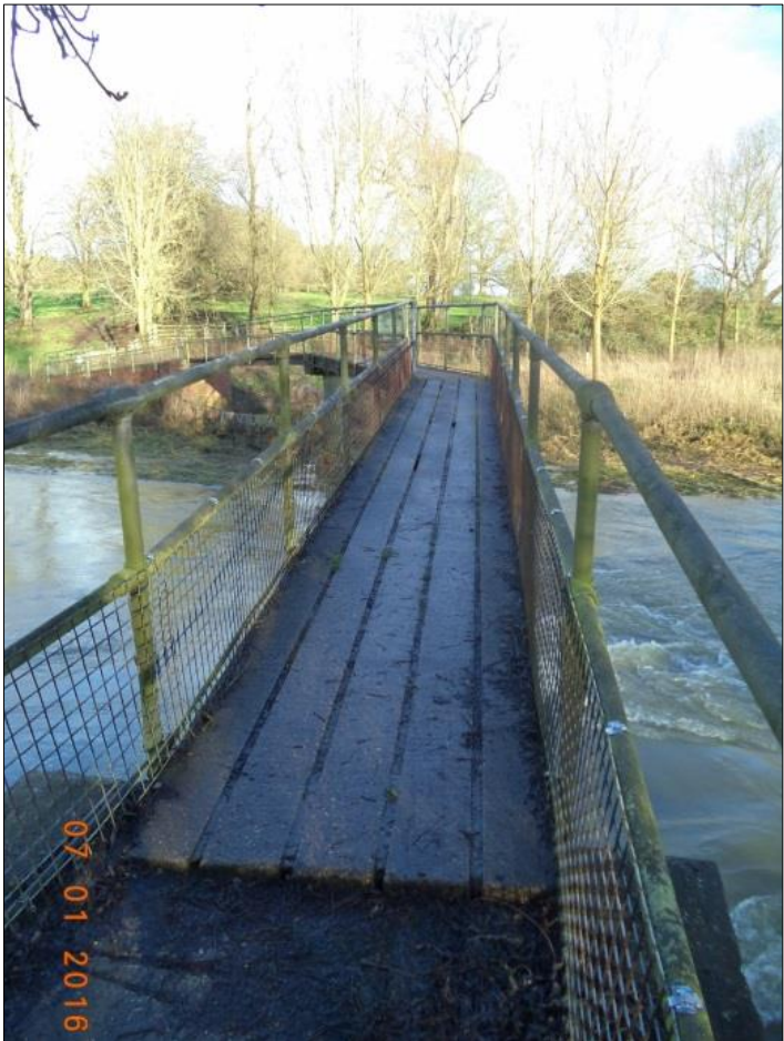
View across old bridge towards Cold Brayfield
