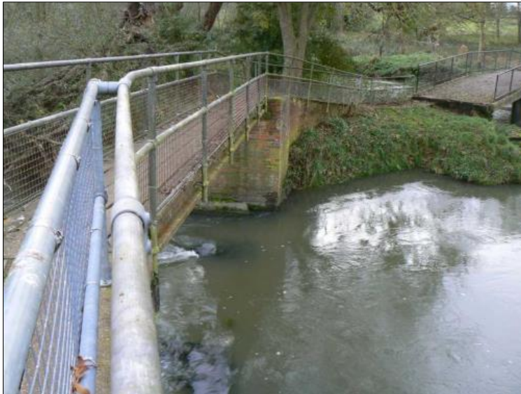
View across old bridge/second bridge towards Newton Blossomville
