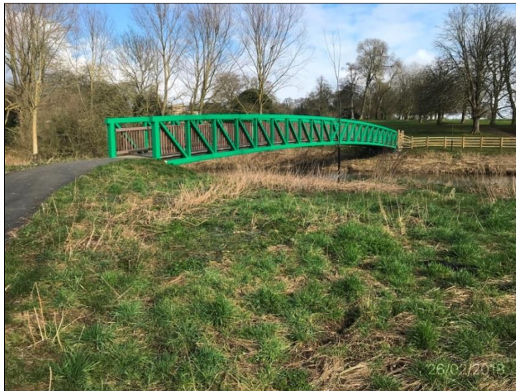
The new Newton Blossomville - Cold Brayfield Bridge
