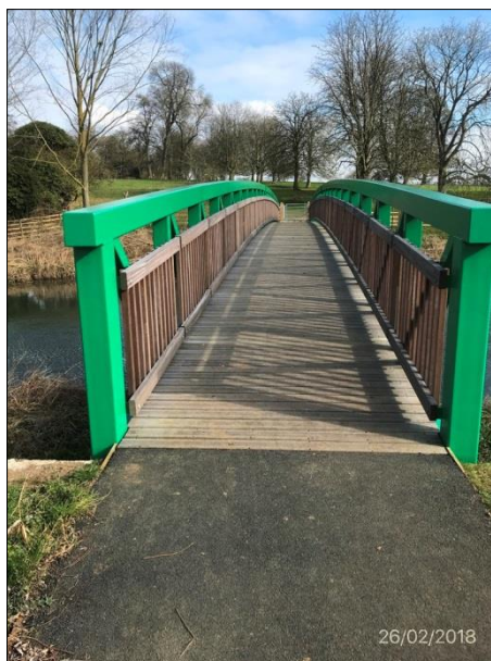
View over new Newton Blossomville - Cold Brayfield Bridge
